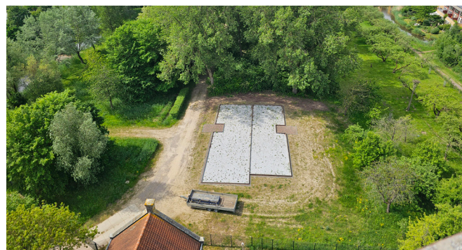
Figure 30: The old sedimentation basins on the Vitens terrain
